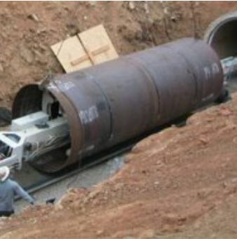
Pipeline Relining $493 million
