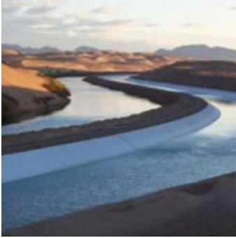
QSA Water Transfer & Canal Linings Hundreds of Millions $
