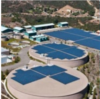
Twin Oaks Valley Water Treatment Plant $179 million
