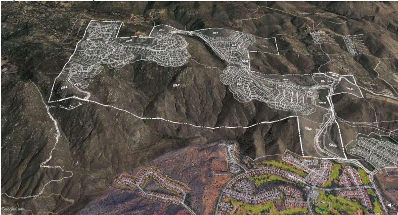
Project aerial view looking west to east
